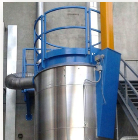
Figure 1: detail of the protection railing
